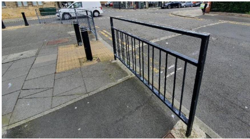
Mismatched and poorly maintained street furniture and surfaces
