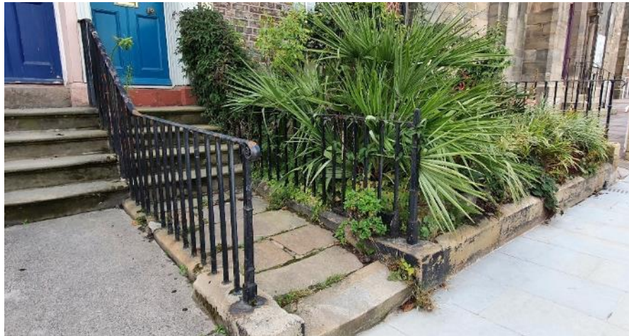
Surviving original railings and green garden
