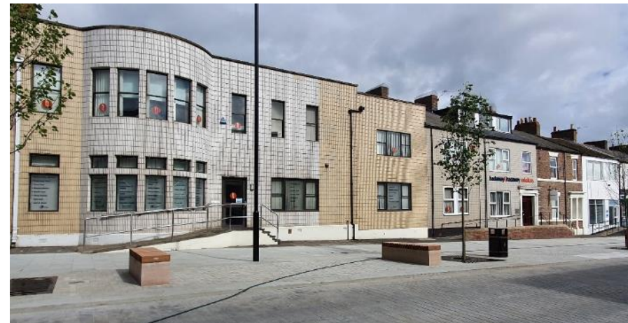
Inappropriate materials on Howard Street
