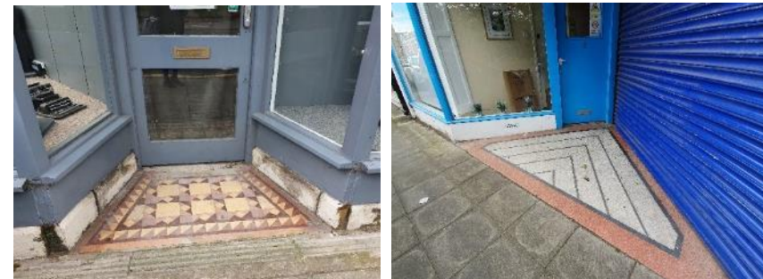
Recessed shopfront doorways with tiled and terrazzo entries on Albion Road
